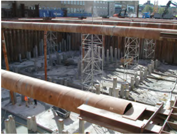
Figure B.5: The excavation after final dewatering in August 2003.
